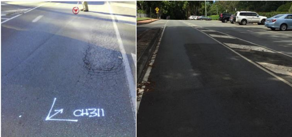
Figure 2G Restoring sealed road condition
